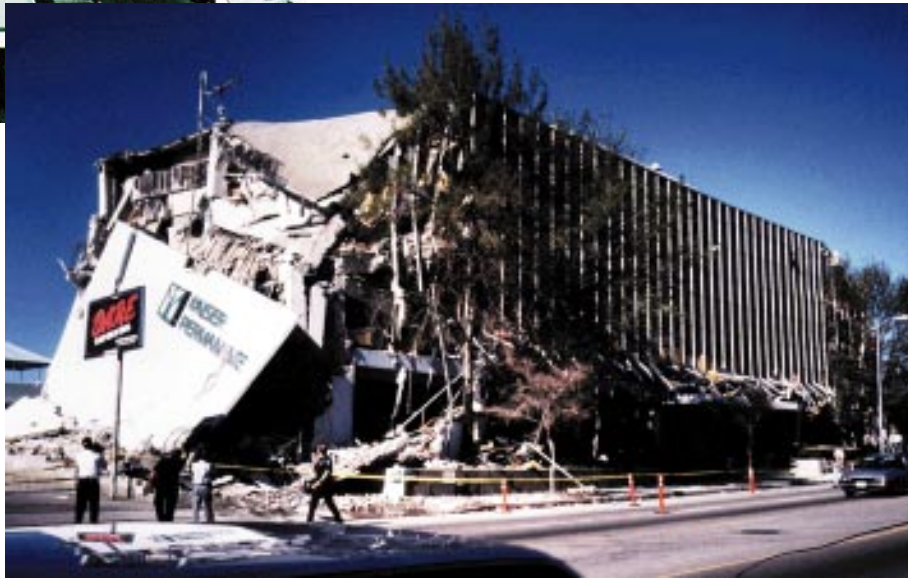
Collapse of this medical building is typical of older concrete building performance.
